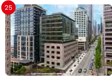
Federal Reserve Building 1015 2nd Avenue, Seattle, WA
